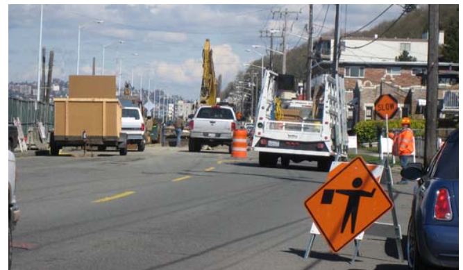
During work hours, flaggers are on site and will help traffic through the construction zone.
