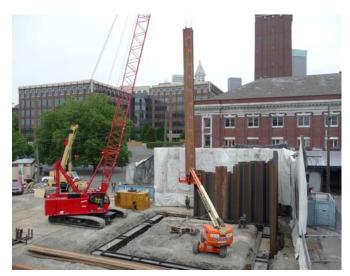
This is an example of sheet piling being lowered in place.
