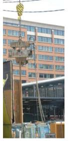
This is an example of how the vibratory hammer and sheet pile suspended from a crane look during pile driving.
