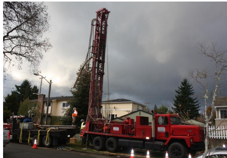
Installation of deep groundwater monitoring well
