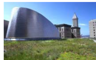
Green roof, Seattle City Hall
