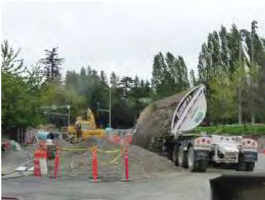
Backfilling with dump truck
