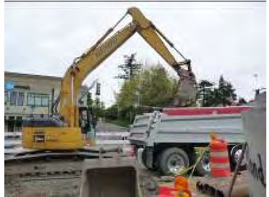
Back-casting to dump truck
