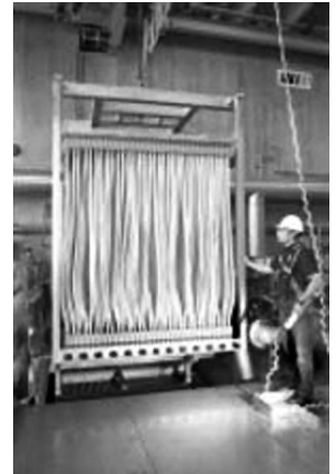
The treatment plant will have large membrane units called cassettes like the one shown above.
