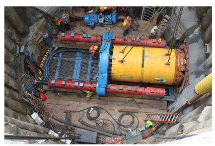
Microtunneling machines like SWIZY help provide safe, reliable sewer service that protects the environment.
