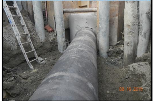
Installed connecting pipe (Queen Anne)
