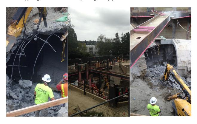
Crews began removing some of the 9- The pipe is being removed to make foot diameter sewer pipe under N.W. way for a new structure to connect Canal St. this week
