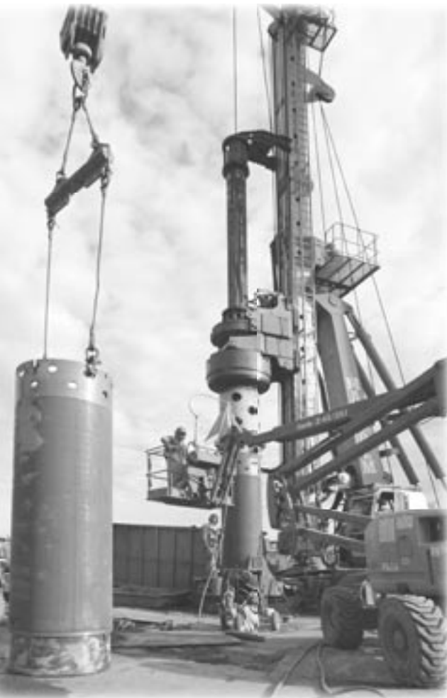
Removing a secant pile casing.
