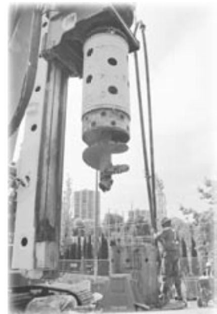
Drilling a secant pile.
