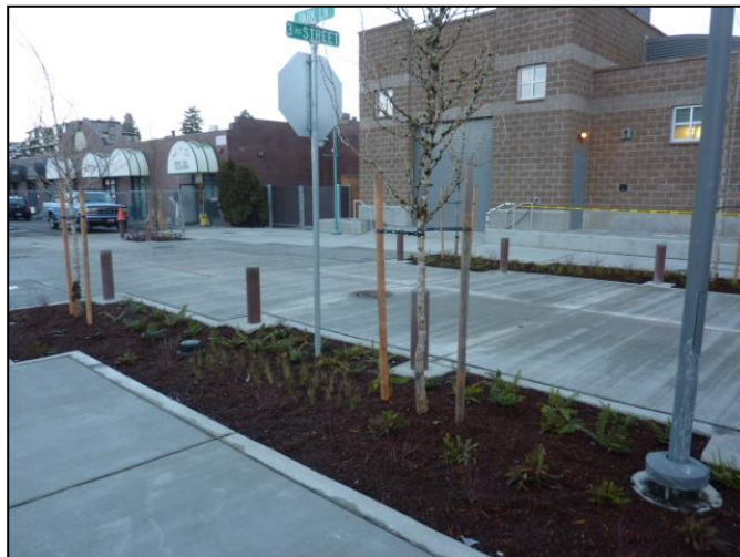
Pump station frontage now includes landscaping, porous pavement and rain gardens to match the flexible street design planned by the City of Kirkland.
