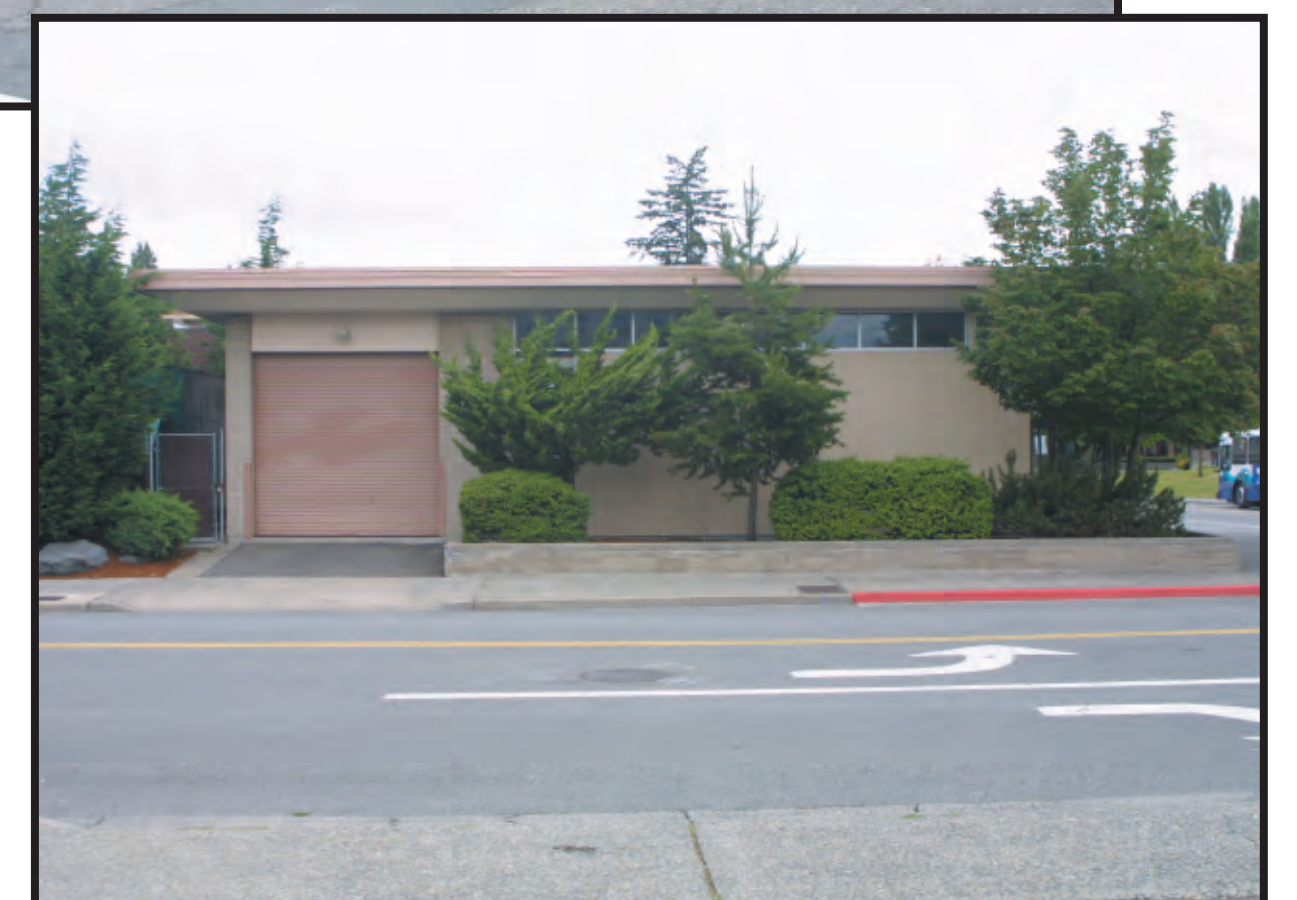
PUMP STATION FROM PARK LANE
