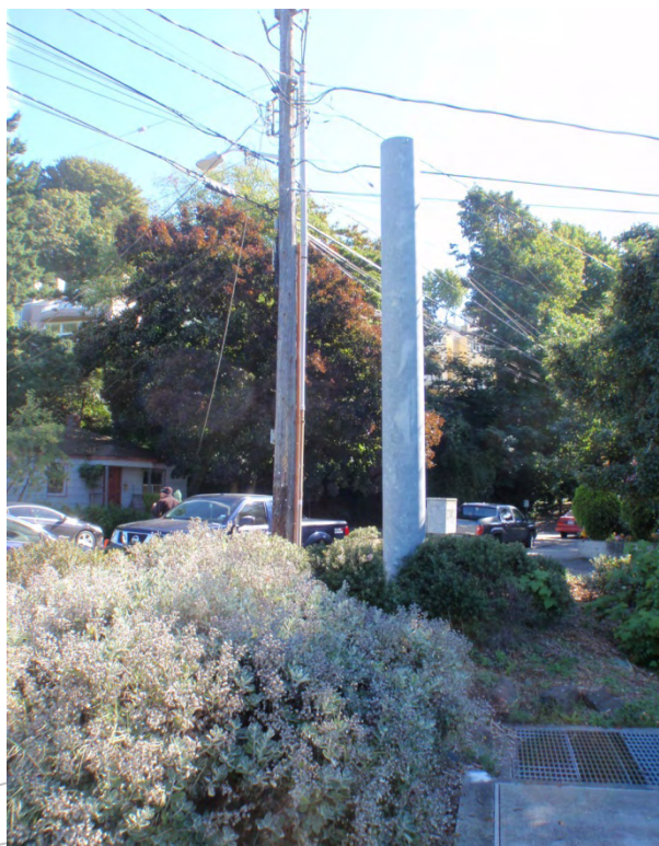
Figure 3: Odor Control System Exhaust Stack.
