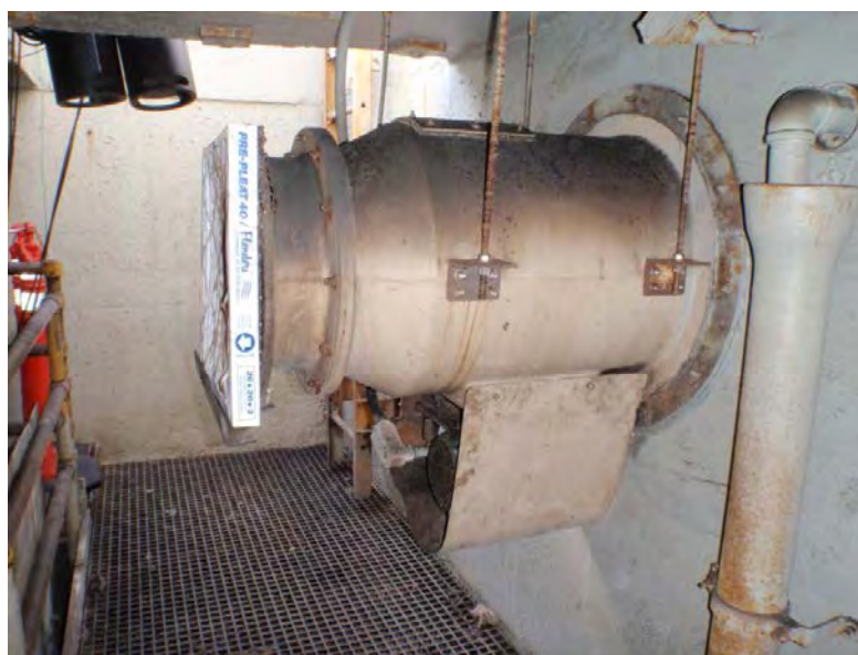
Figure 5: Wet Well Exhaust Fan (mounted on north wall, with filter).
