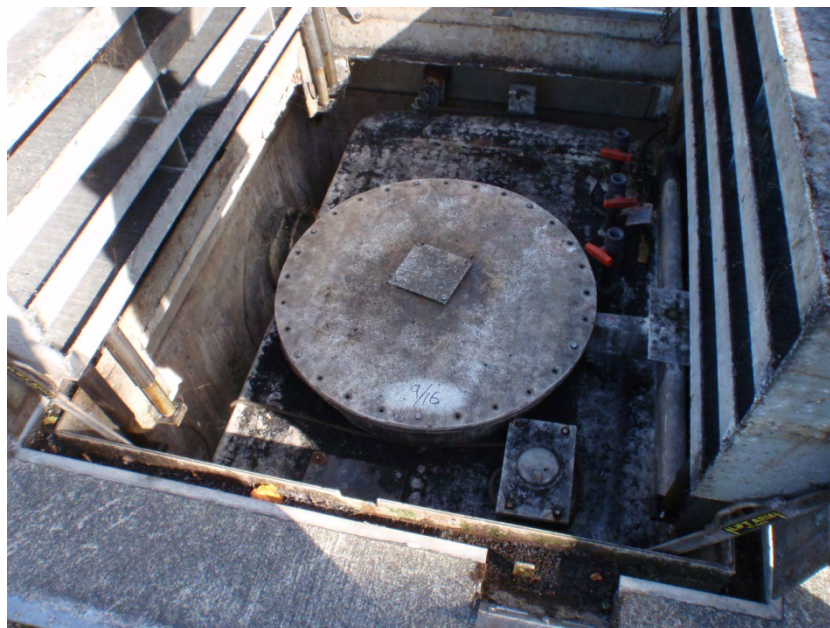
Figure 4: Odor Control Carbon Vessel.
