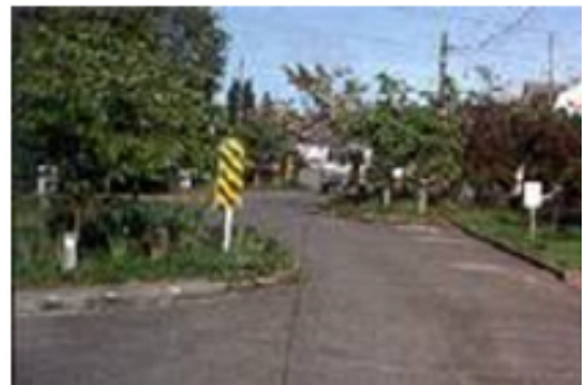
(SDOT requires object marker signs at the Beach Drive Southwest mid-block curb bulbs)
