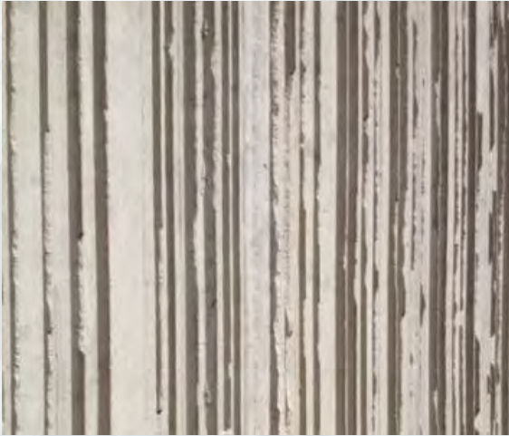
Corduroy textured concrete
