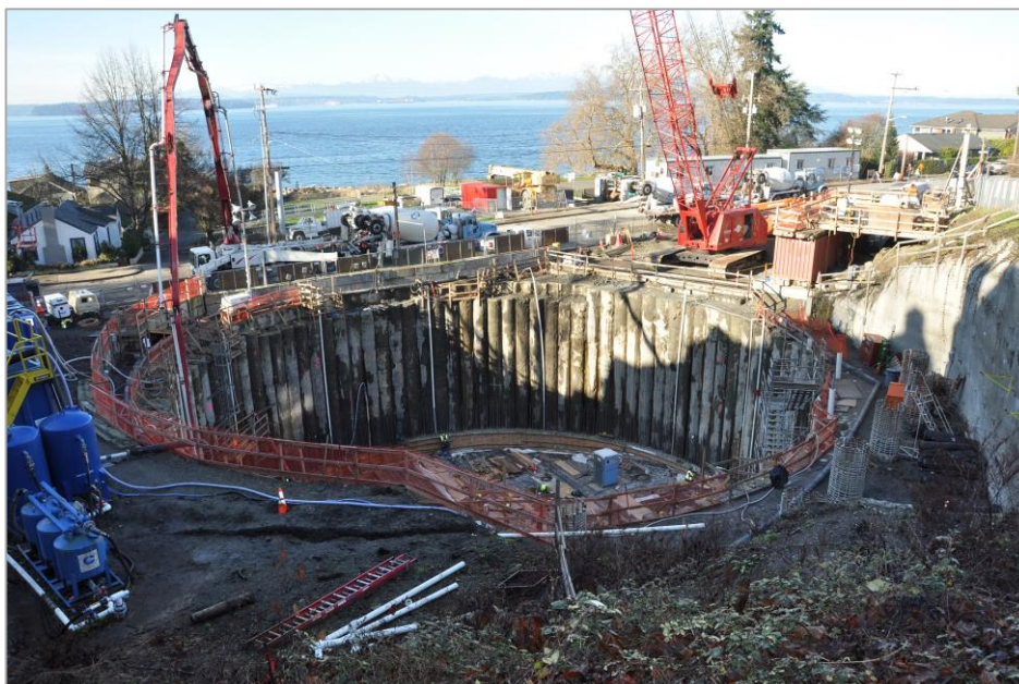
King County contractors recently finished the first concrete pours in construction of the underground storage tank.
