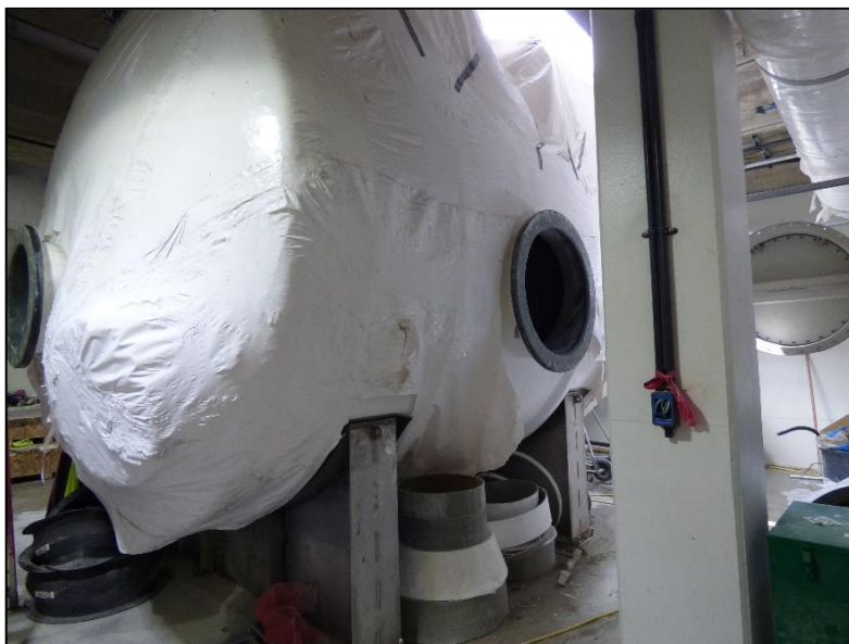
Large tanks inside the odor control room hold carbon filters to reduce odors and maintain air quality.
