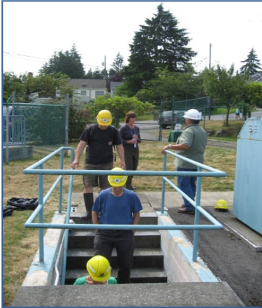
Neighbors tour the inside of the pump station
