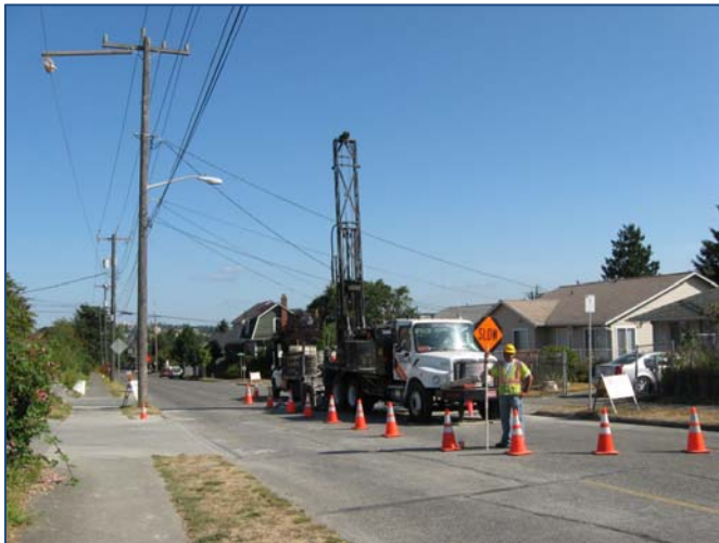
Truck-mounted drill rig
