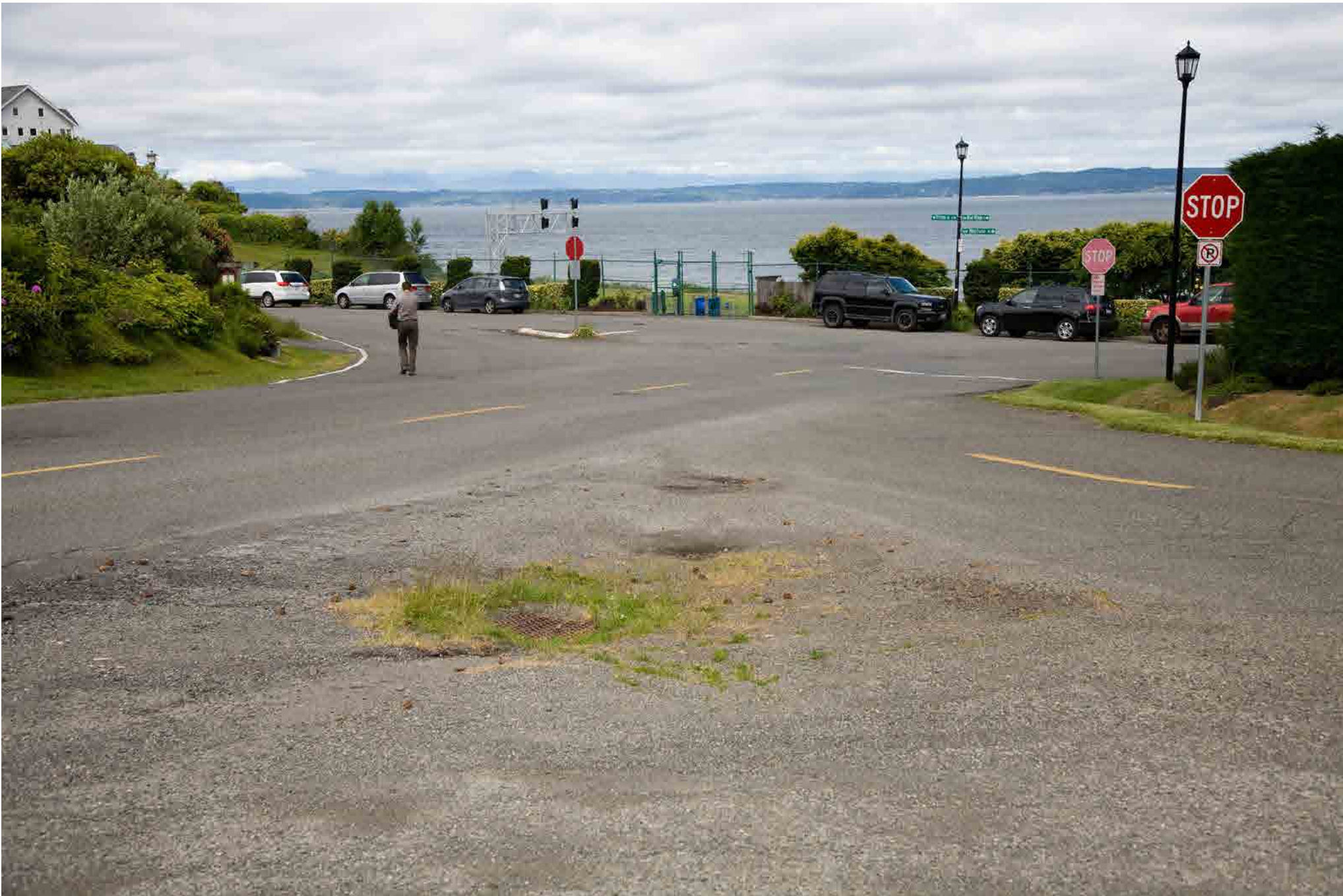
Looking Northwest toward Blue Ridge Park
