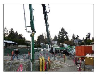
A pump mounted on a truck pours concrete deep in the excavated area to form the base of the CSO tank.
