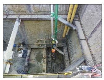
Crews direct the concrete pump to pour concrete into the rebar form, which will become the base of the CSO tank.
