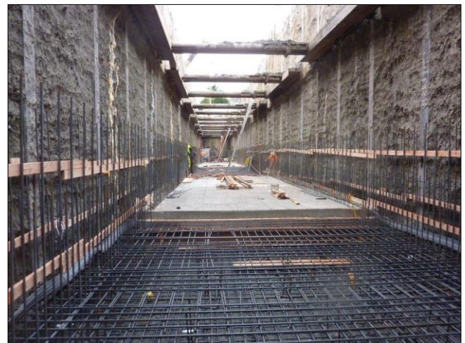
Views from inside the CSO tank as it is being built.
