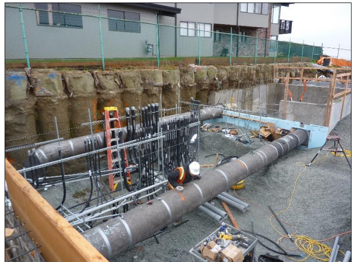
Electrical lines are being installed for the mechanical/electrical building.
