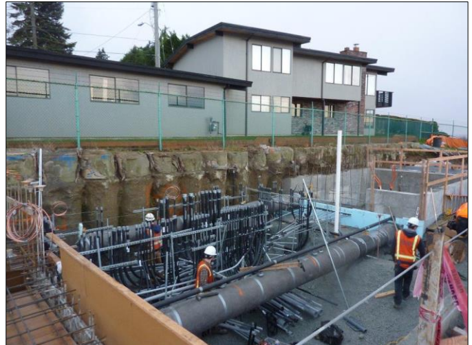
Crews continue to install electrical lines for the mechanical/electrical building.
