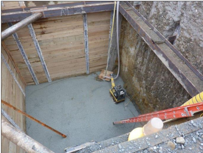
A view inside the excavation area for the 48b structure.
