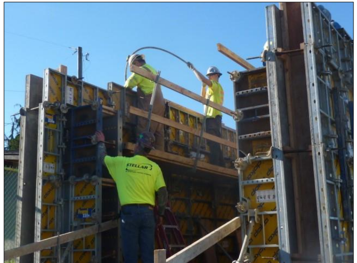
Crews forming the walls for the mechanical/electrical building.
