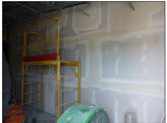
Inside the mechanical/electrical building crews have installed drywall.
