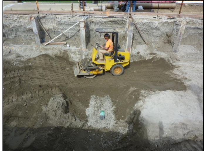
Crews continuing to backfill the area above the CSO tank.
