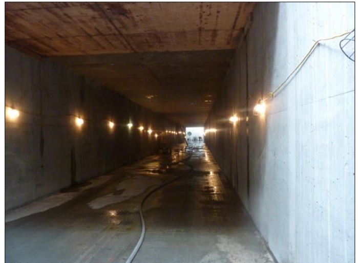
A view inside the underground CSO tank.
