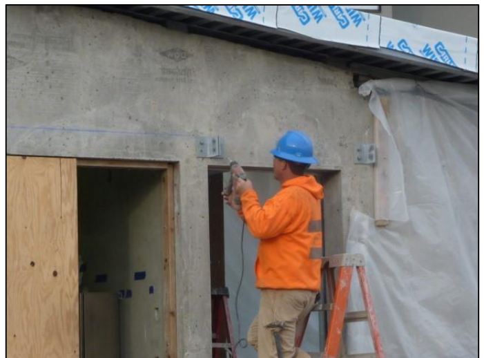
Crews continue work on the Mechanical/Electrical Building.
