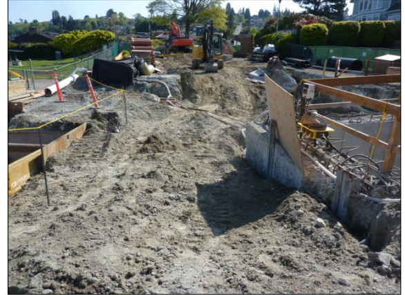
Crews continue to backfill the area above the CSO tank.
