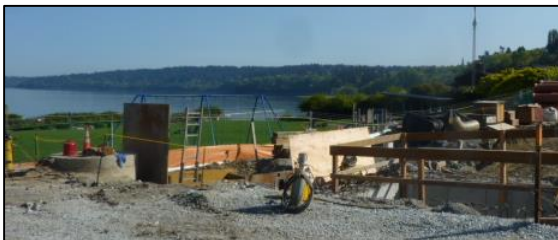
The construction site on April 20, 2015.
