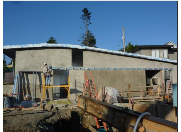
Crews continue work on the mechanical/electrical building.
