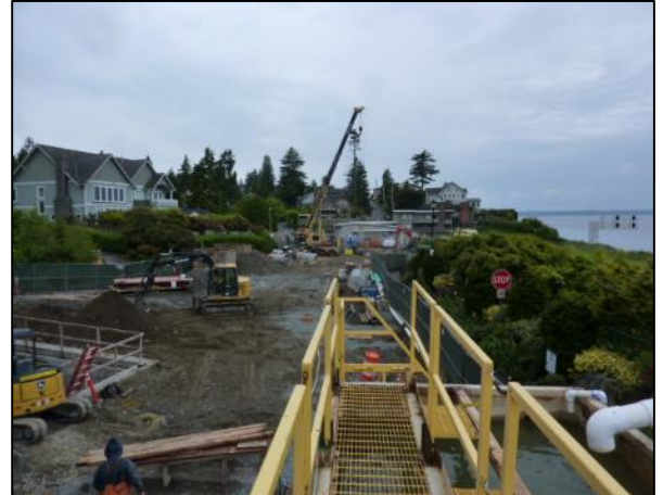
Construction site as of June 1, 2015.
