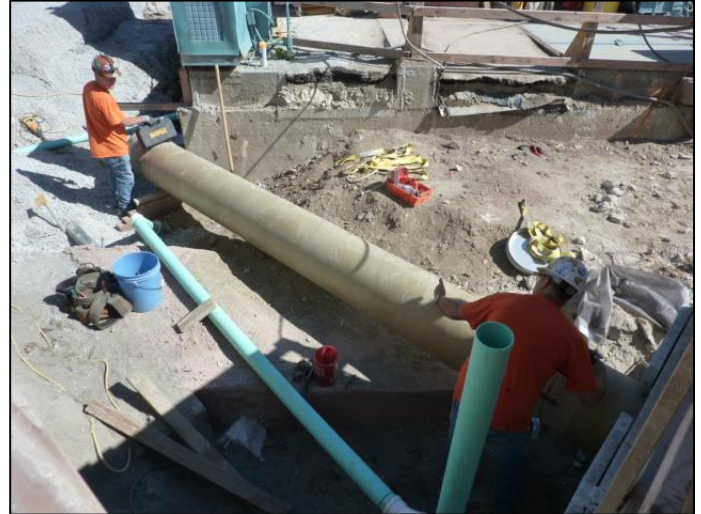
Crews installing new fiberglass pipe to connect wastewater infrastructure.
