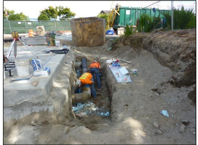
Crews connect pipes to the CSO flushing vault.
