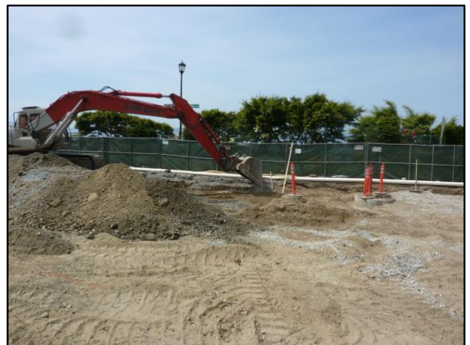
Crews level out the site to prepare for paving.
