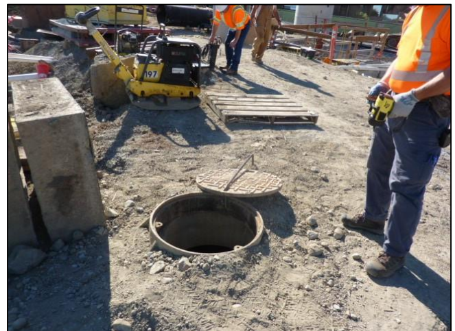
Sitework to connect wastewater infrastructure and installation of new manholes.
