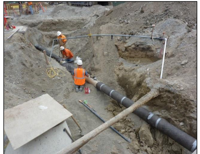
Crews work on the new wastewater infrastructure on-site.
