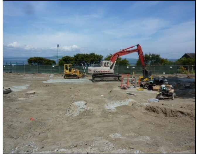
The construction site on July 21.
