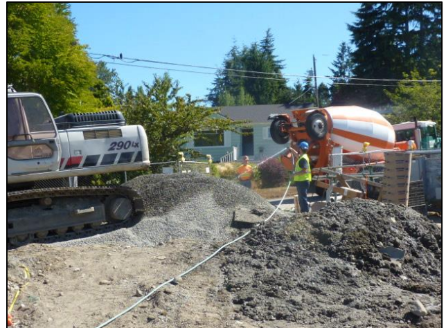
Crews using water to control dust on-site.
