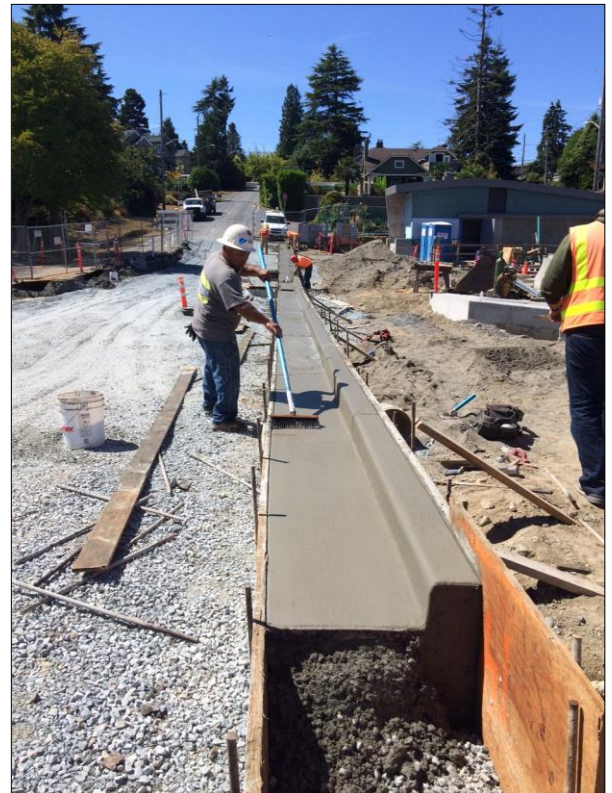
Crews install new curbs in preparation for paving next week.
