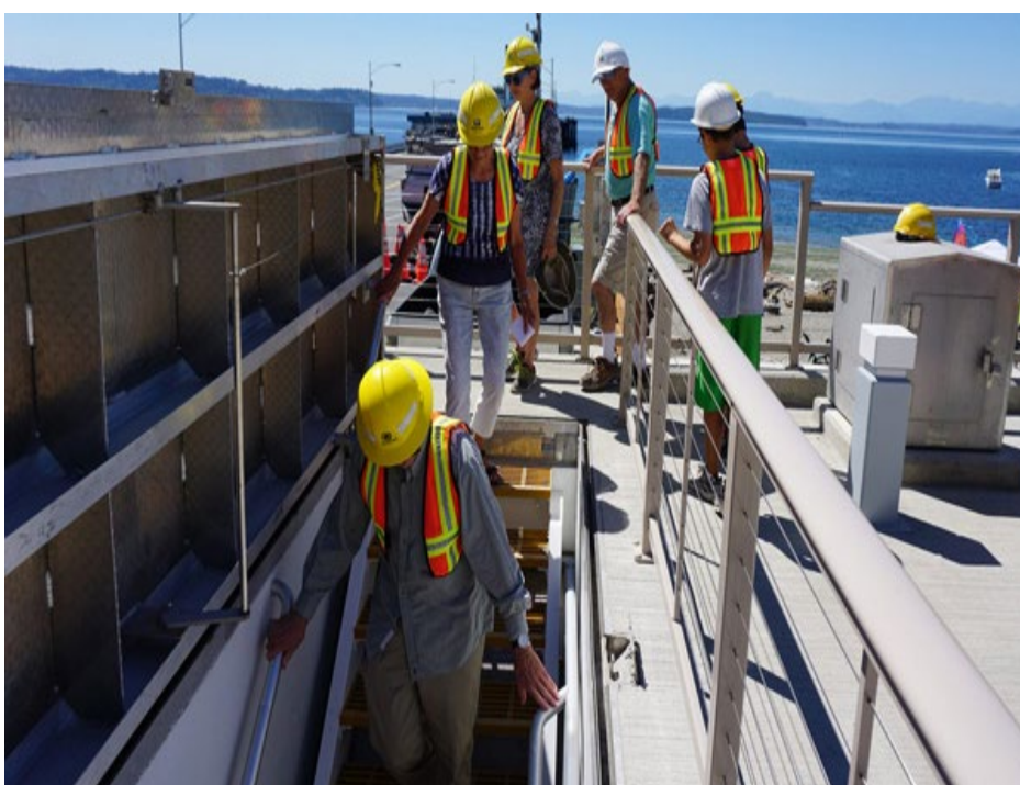
Tour of the Barton Pump Station (underground)
