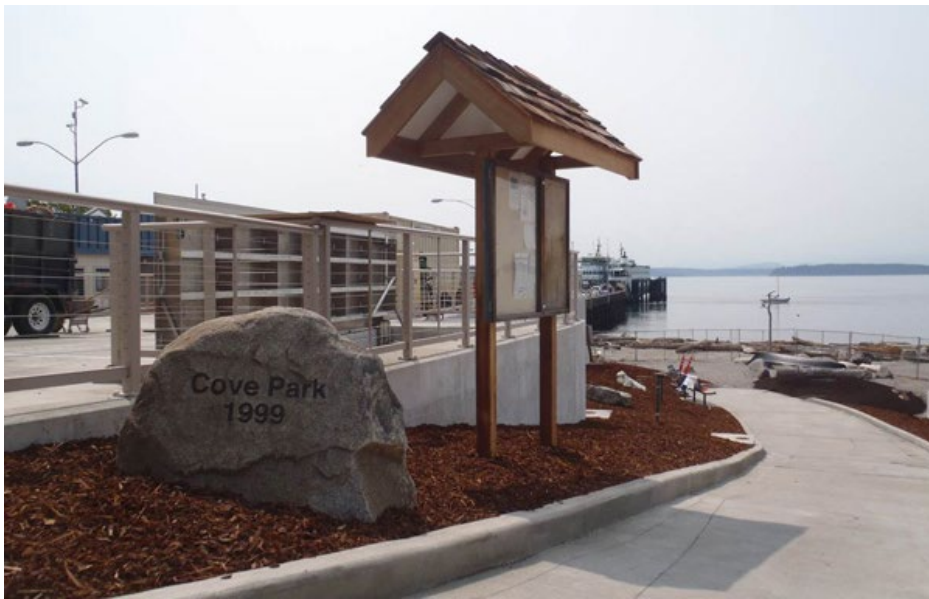
New kiosk located next to Barton Street Pump Station
