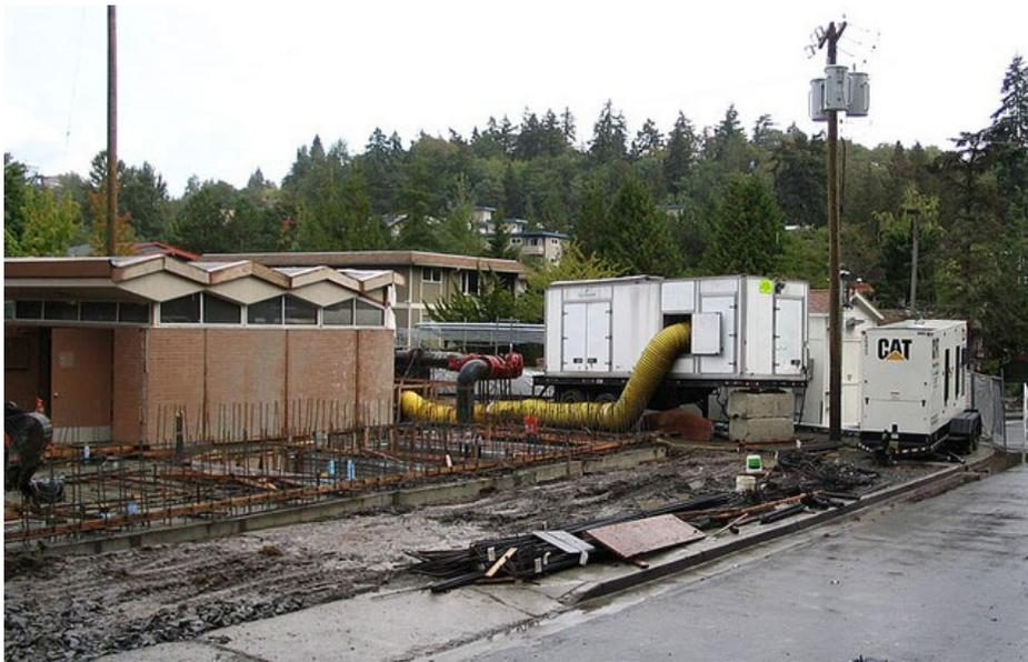
Oct. 2009. The old pump station (left) prior to demolition, temporary pump facility (on trailer), and foundation for new generator building.
