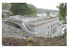
The outlet regulator is designed with an environmentally friendly "green roof" that collects and reuses stormwater runoff and keeps it from entering the combined sewer system.
