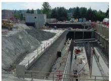
The North Creek Storage Facility, which is designed to temporarily contain potential wastewater overflows, particularly during peak storms, will help to eliminate overflows into Lake Washington near Kenmore.
