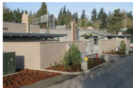
Sweyolocken Pump Station, 3100 Bellevue Way S.E., Bellevue
