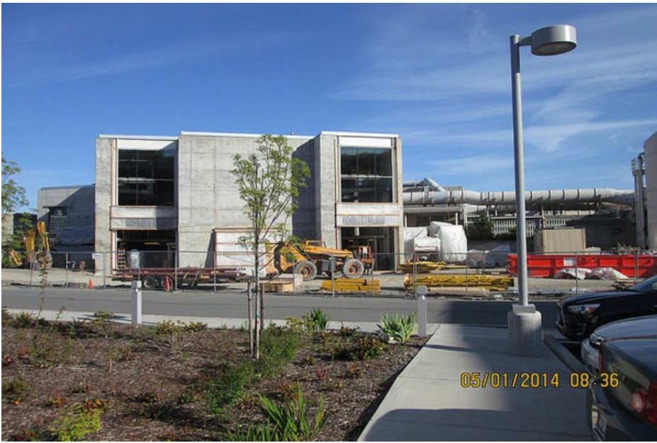
Screenings handling building
