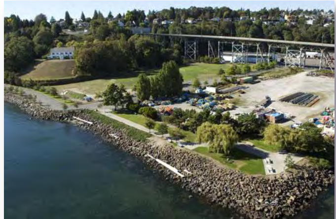
Storage tank site location
