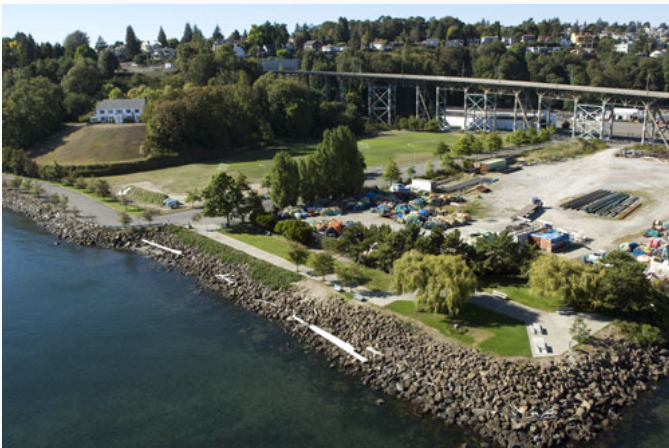
Storage tank site location in the West Yard, at right
