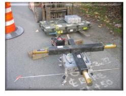
Tracking devices at the surface track the drill bit location during the initial bore
