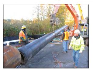
Heavy equipment is used to lift the pipe and pull it through the prepared bore hole
