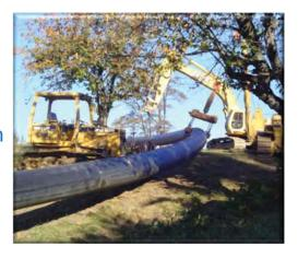
The pilot hole is then enlarged to the final pipe size using a reamer. The drilling mud excavated in this step is collected and recycled.
