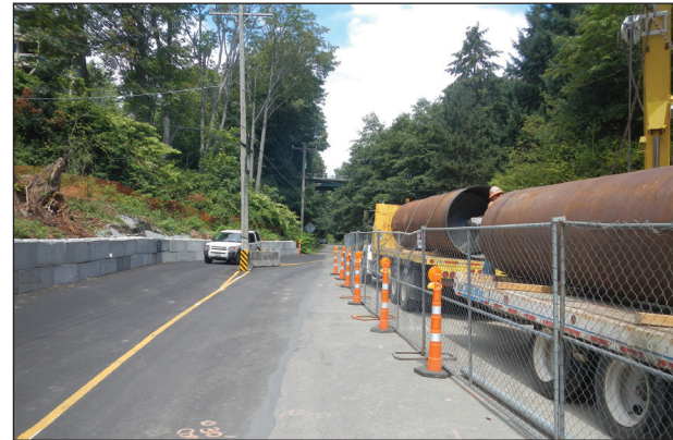
Conductor casings are used to protect the hillside where the pipeline enters and exits
