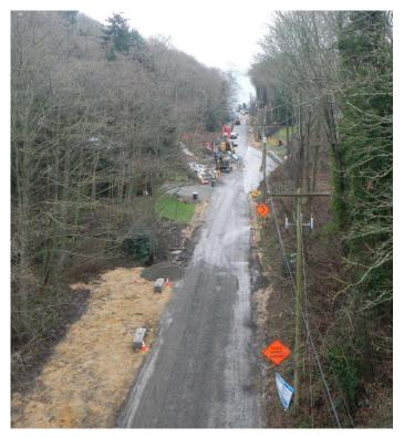
pipeline. This structure, located on 32<sup>nd</sup> Avenue West near the drill pit, will direct excess flows from the existing sewer system to the new pipeline. Next week, crews will install shoring for the new diversion structure. The shoring system used for this structure, like the system used for the drill pit, does not require vibratory methods to install.
