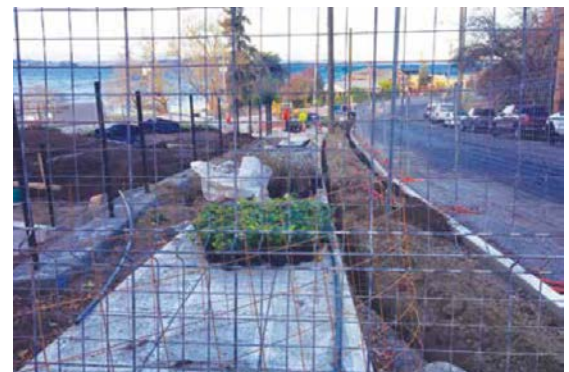
Install security fencing around the project site.
