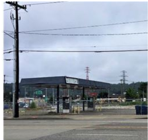
To prepare for construction, crews will demolish the fuel island.
